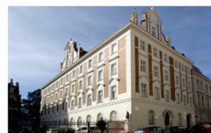
Picture 4: Monastery Building After Renovation, ©Schöberl & Pöll GmbH
